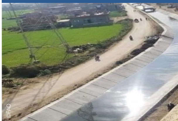
FIGURE 20. Lining main irrigation canals
